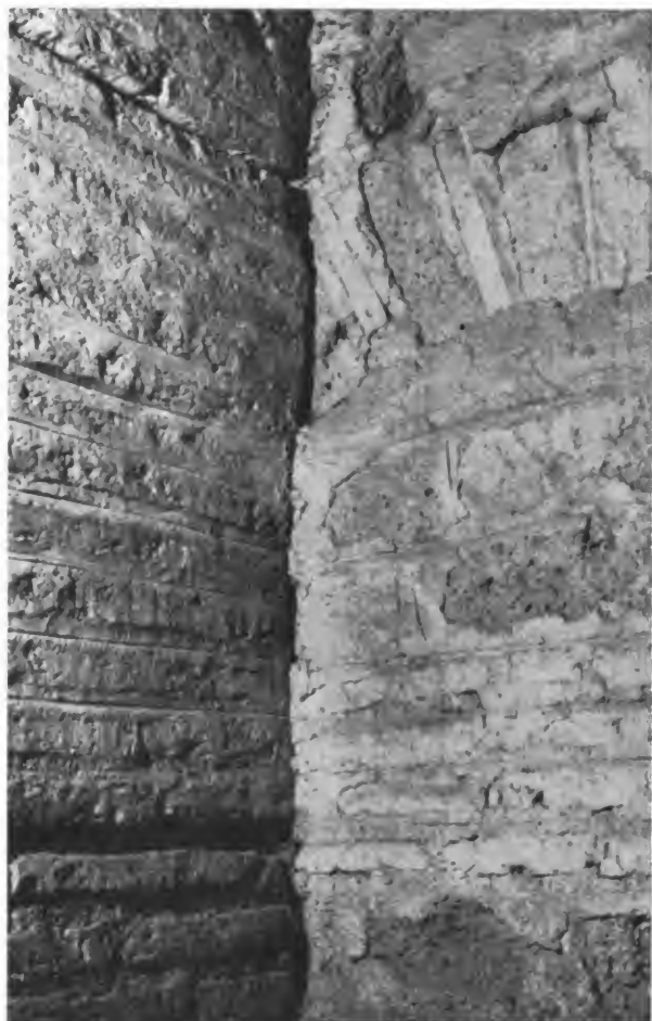
Fig. 228 — S. Maria in Cosmedin. Correspondence of the diaconia opening, the campanile, and the wall which seals the opening (Photo: Corbett).
